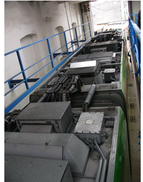
Mechanism for regenerative brake on the roof of a Škoda Astra tram
